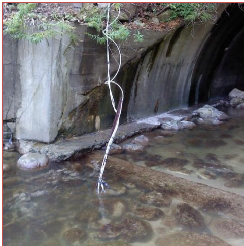
Gully Creek – low flow
