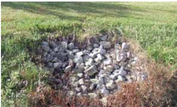
BMPs like rock chutes help improve water quality.
